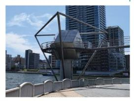
Reiganjima Tide Station opened at the mouth of Sumida River in 1873. It was a water level observatory to designate the altitude standard. The average water level measured with the water level marker of this tide station was set as standard (altitude 0 meter) and was used to designate the altitude of the Japanese datum of leveling (Nagatacho, Chiyoda City). A symbolic observation pillar stands at the site of the former tide station.
